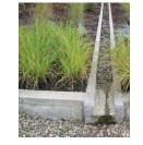
**Bio-swales:** Bio-swales (or rain water swales) collect rain and water that runs off of the roof and pavement, an impervious surface, and cleans it by filtering it through water quality plants before it returns to the creek and watershed.
